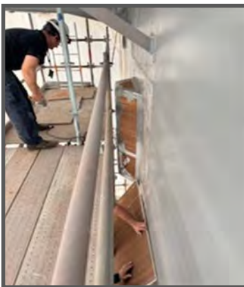
Staging and enclosure made in preparation for patch installment.
