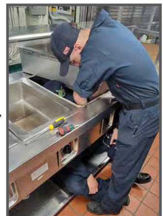
FN Jace Peterson preparing to mount a new steam table. (Photo by Rizalito Antonio.)
