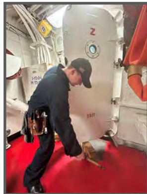
DC3 Jake Andersen using a DC Wedge to lift door for hinge pin replacement of QAWTD 2-173-2 (Photo by Ramir Pulido.)
