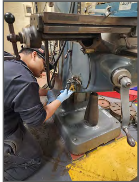
MR3 Robert Figueroa inspecting the lubricating filter before installing the lubricator holding unit for the Bridgeboard Milling Machine.
