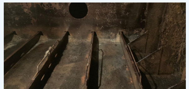
Ballast tank coated in S2S
