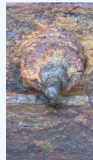
Steep Creek Bridge - Uncoated
